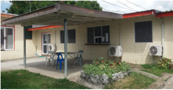
Front view- additional room with information window.
