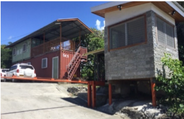
Security guard room and boom gate at the entrance to EO.
